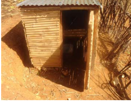
Part of the village's environmental focus is on sanitation improvement. Household latrines like this one are made of bamboo.
